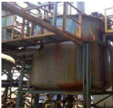
Photograph of 2 tonnes/ batch leaching reactor
