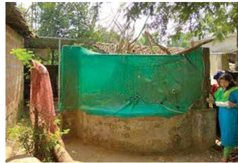
A perchlorate contaminated community well closed by health department in Keezhmad panchayat, Aluva.
